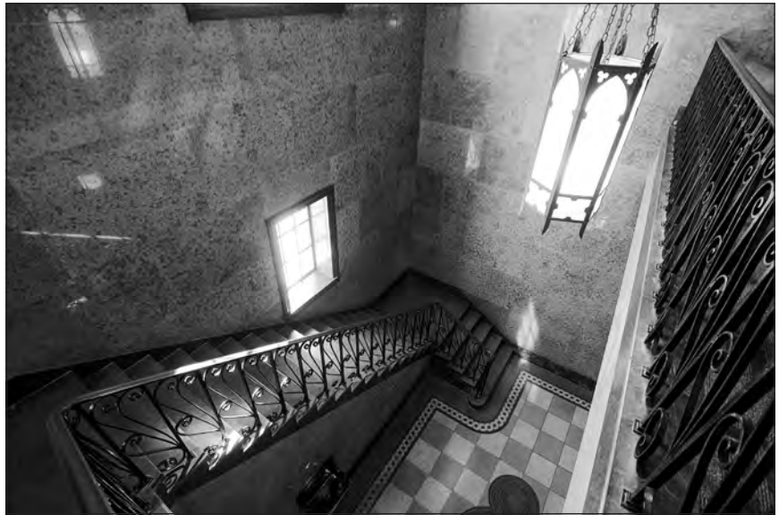
The original granite walls and floors, as well as the original iron stair railings, make for an elegant entrance from the foyer to the renovated auditorium.
